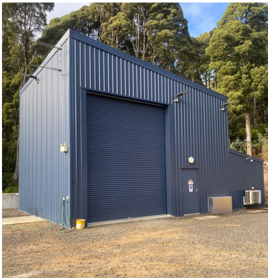
Scottsdale power station
