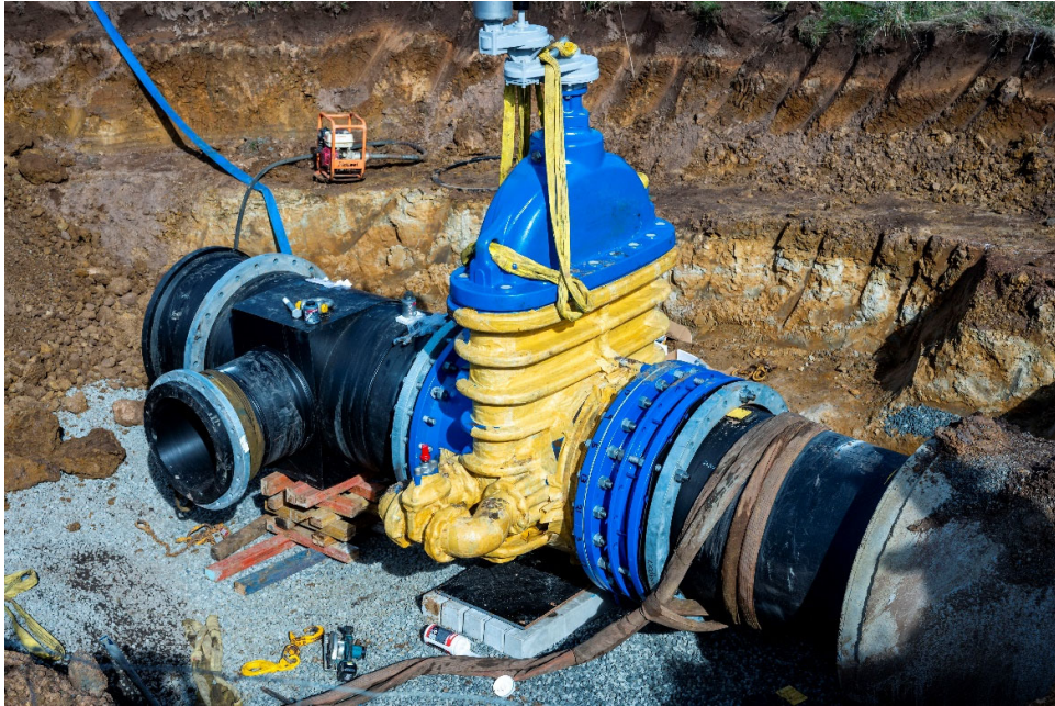
Valve Installation works
