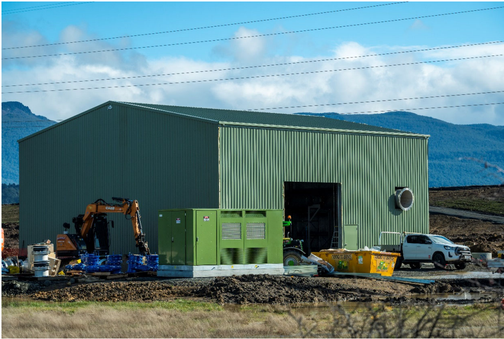
Poatina Pump Station
