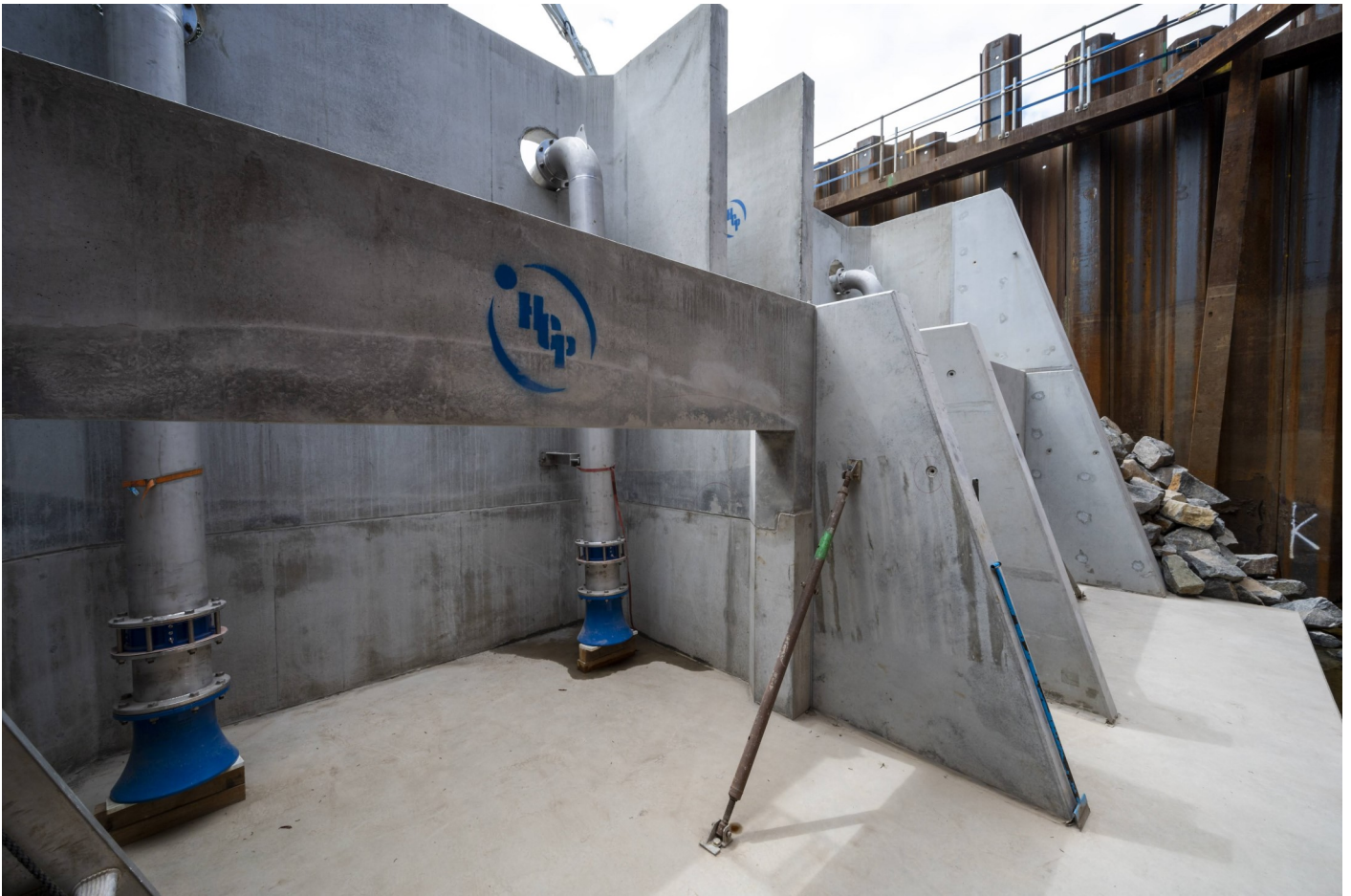
Picture: Construction work continues on the Don Irrigation Scheme
