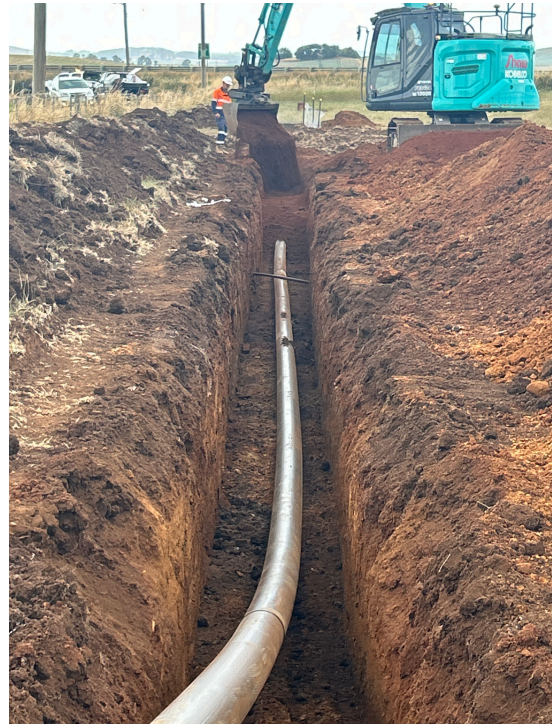
Pipe being laid near Sassafras as part of the augmentation
