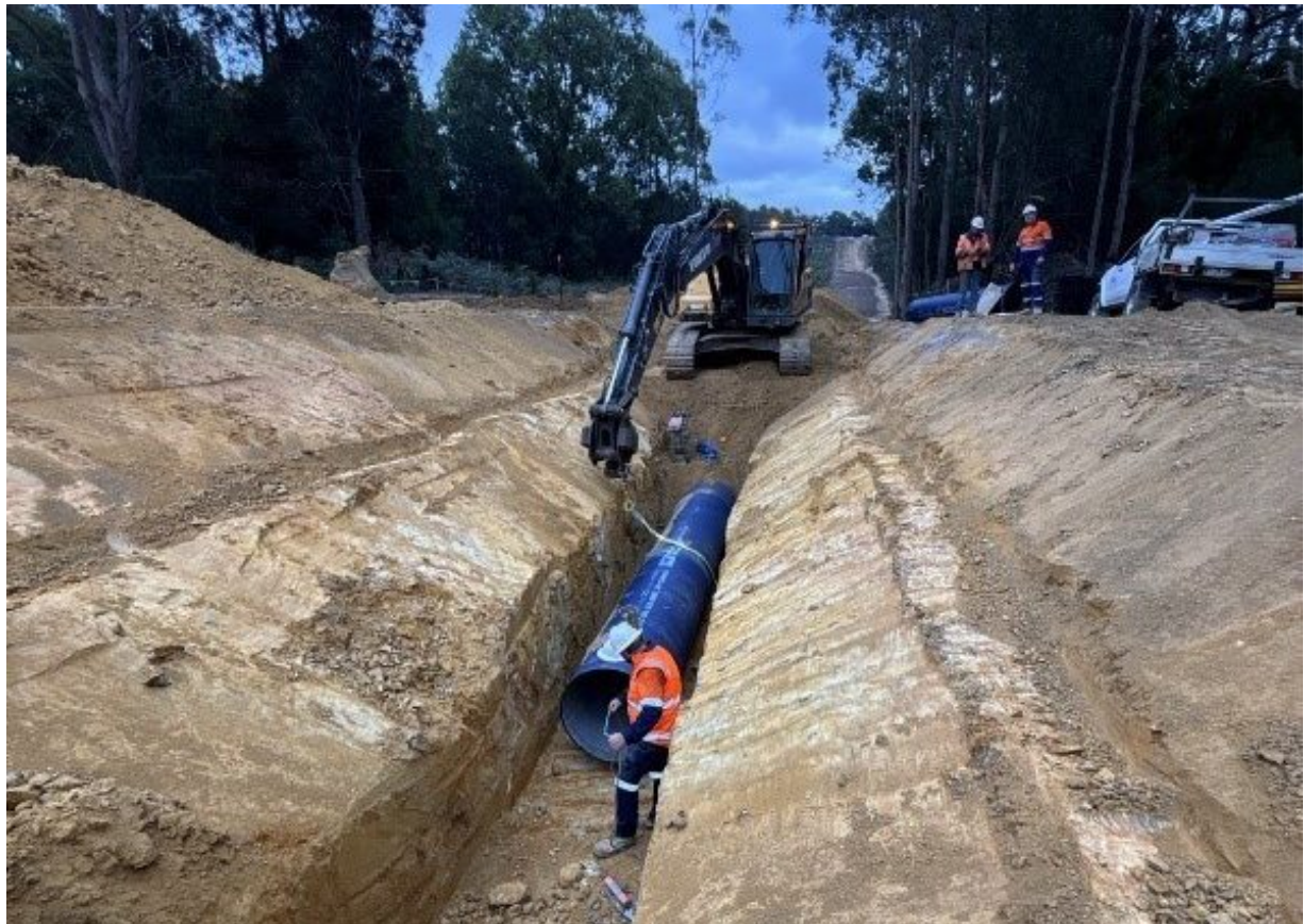
Over 30km of pipe is now in the ground on SWISA
