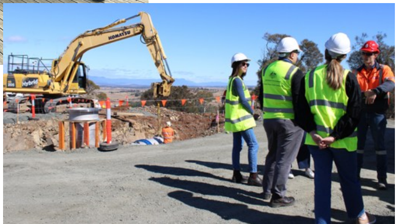
NWG representatives learn about the Northern Midlands Irrigation Scheme at the Valleyfield header tank construction site
