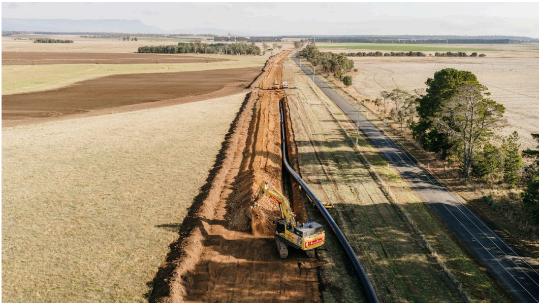
Figure 1 - 147km of the 152km pipeline has been installed.
