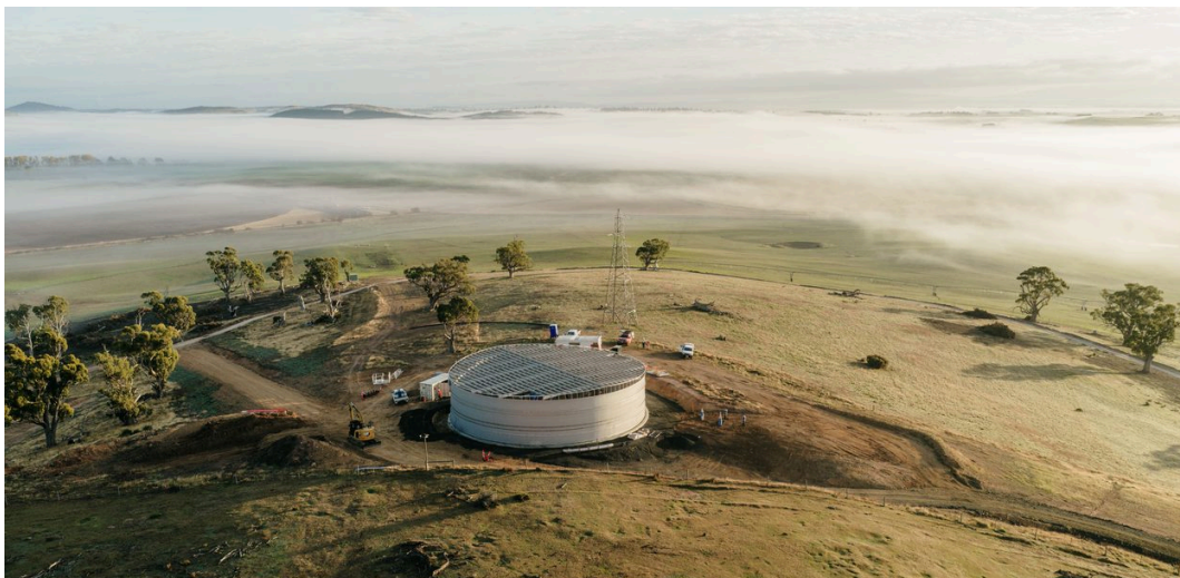
Figure 2 - The 3.45-megalitre Poatina Balance Tank is now almost completed.
