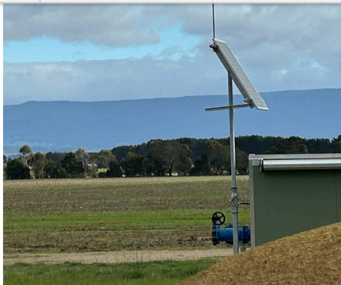
Figure 3 - The final few property outlets are being installed across NMIS.
