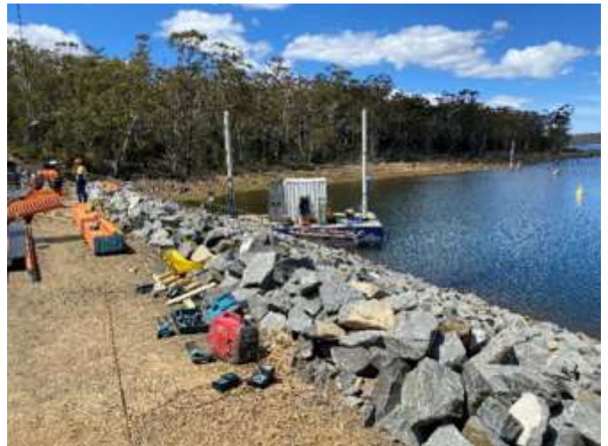
New rock armour on the Lake Leake spillway upgrade
