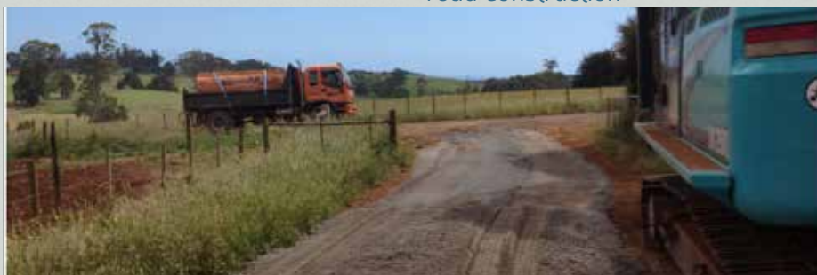
Figure 4: Commencement of access road construction
