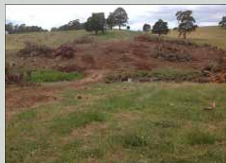
Figure 3: Dam post timber removal dam site
