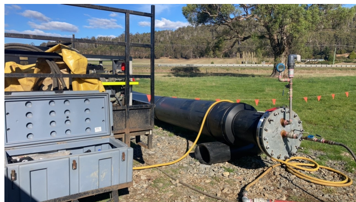
Pressure testing at Quamby
