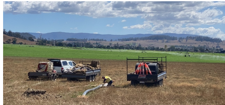
Preparing to test new connection at Caveside
