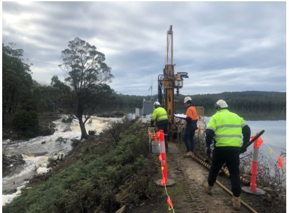
↑ Drilling works at Lake Leake
