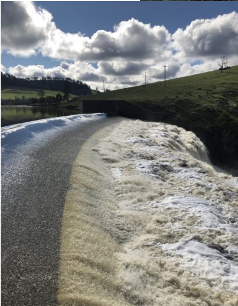
Craigbourne Dam in flood ↑
