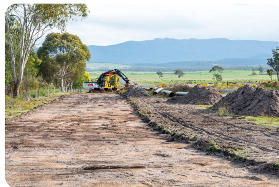
Topsoil stripping - Barton Road
