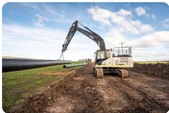
Pipe welding - Ashby Road
