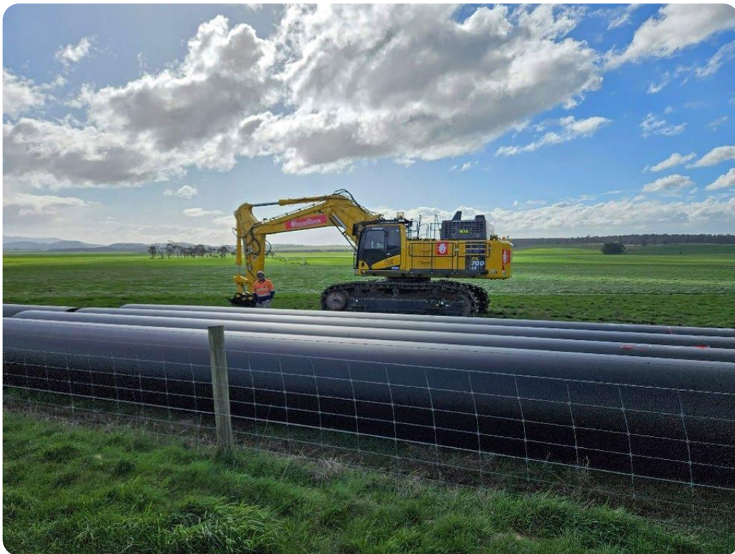
Pipeline construction, NM1 Zone, Cressy
