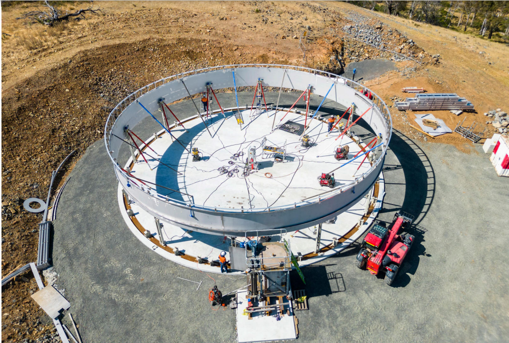
Figure 2 - Valleyfield balance tank construction
