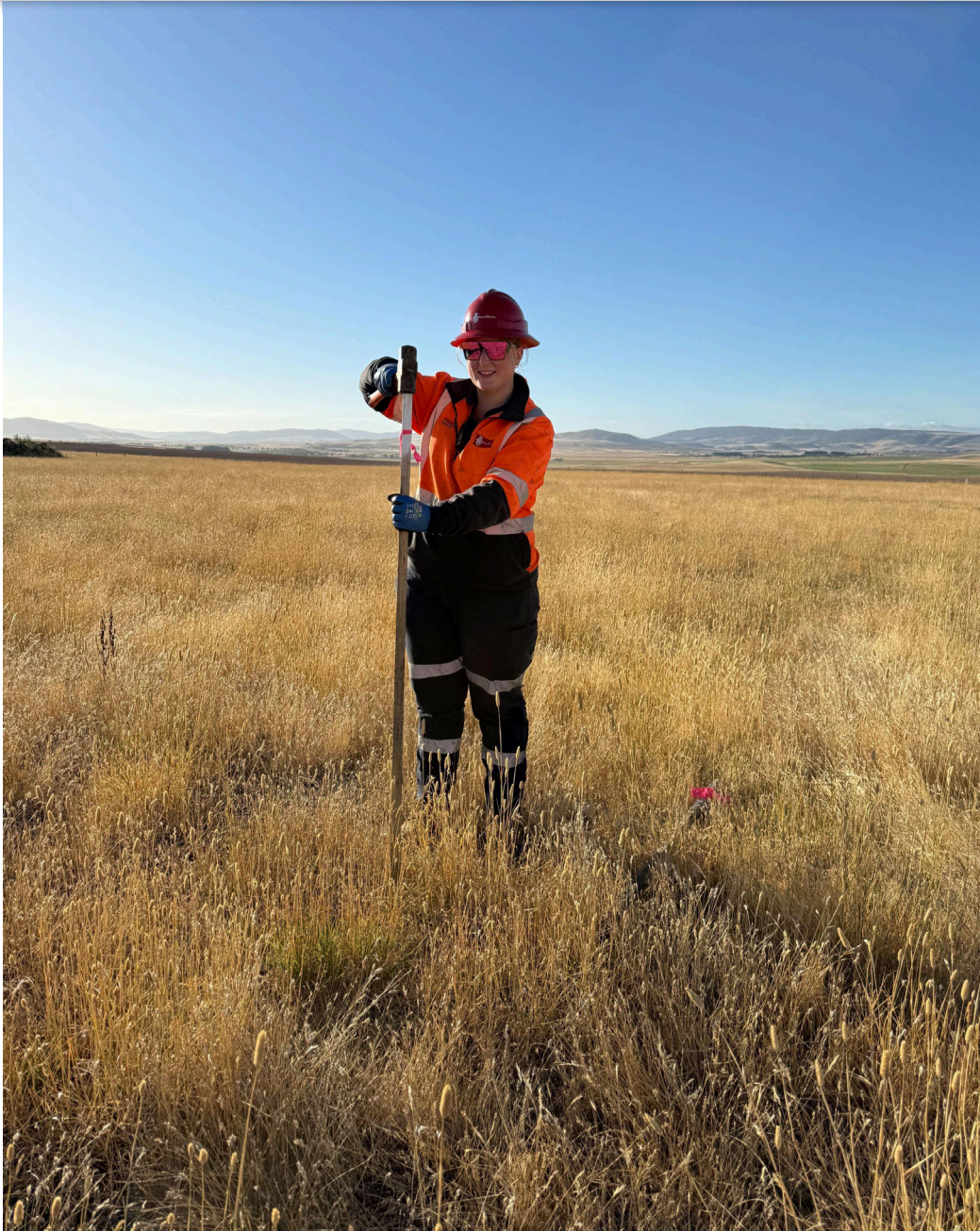
Figure 3 - Jen demarcating the construction corridor
