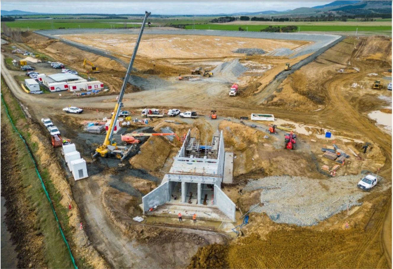
Poatina Buffer Dam and inlet structure in foreground
